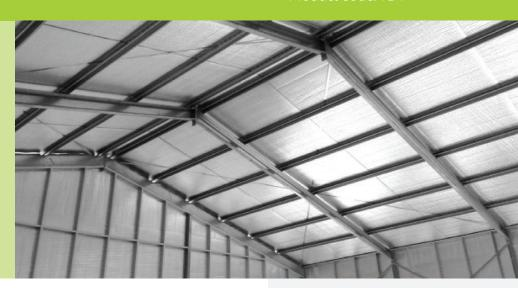
ThermalLiner™ is an Extra Heavy Duty three-in-one reflective insulation, thermal break and Class 2 Vapour Barrier. ThermalLiner™ is suitable for use in roof, wall and floor applications. Designed to manage heat gain and heat loss, ThermalLiner™ offers superior thermal performance to conventional insulation, and reduces thermal bridging and conductivity between building elements.
